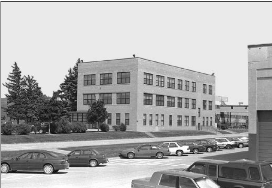
Plate 97. Oblique view of the A Building (first SAC Command Headquarters). View of July 1999. Photograph, K.J. Weitze.
