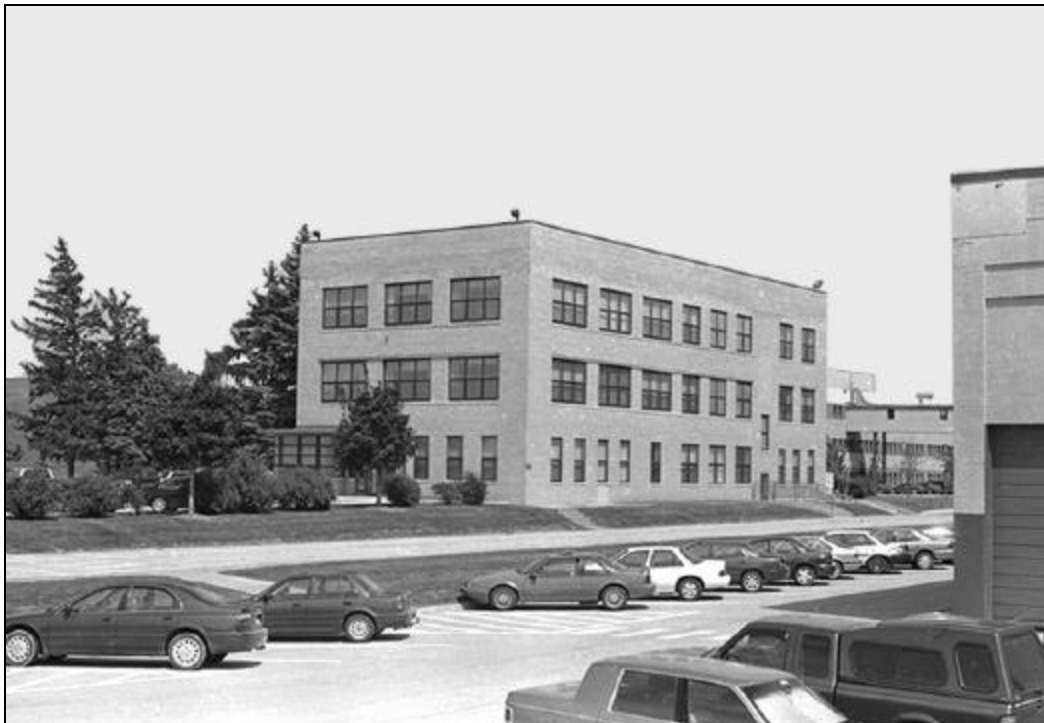
Plate 97. Oblique view of the A Building (first SAC Command Headquarters). View of July 1999. Photograph, K.J. Weitze.
