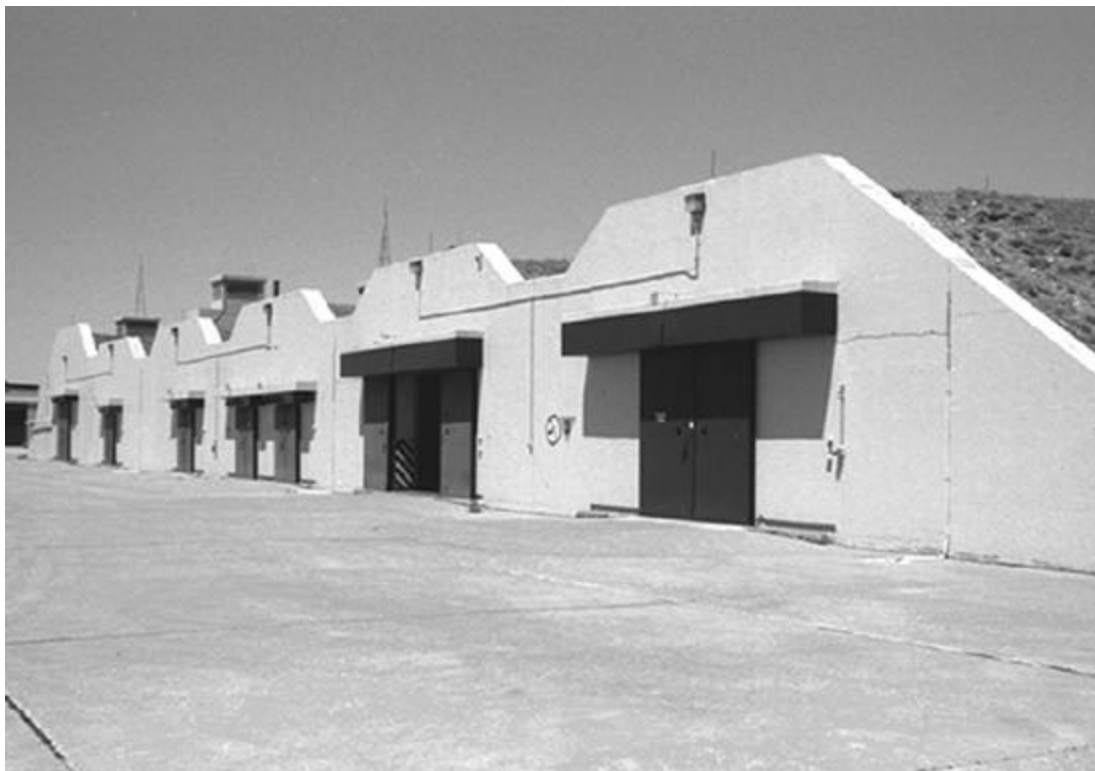
Plate 98. Black & Veatch. Plant I (A) in the Q Area at Ellsworth Air Force Base. View of 1995. Courtesy of Mariah Associates, Inc.
