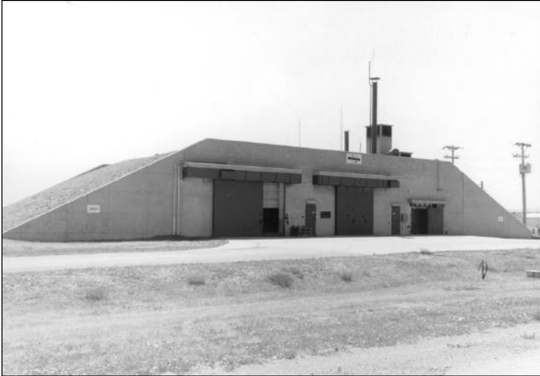
Plate 99. Black & Veatch. Plant II (B) in the Q Area at Ellsworth Air Force Base. View of 1995. Courtesy of Mariah Associates, Inc.
