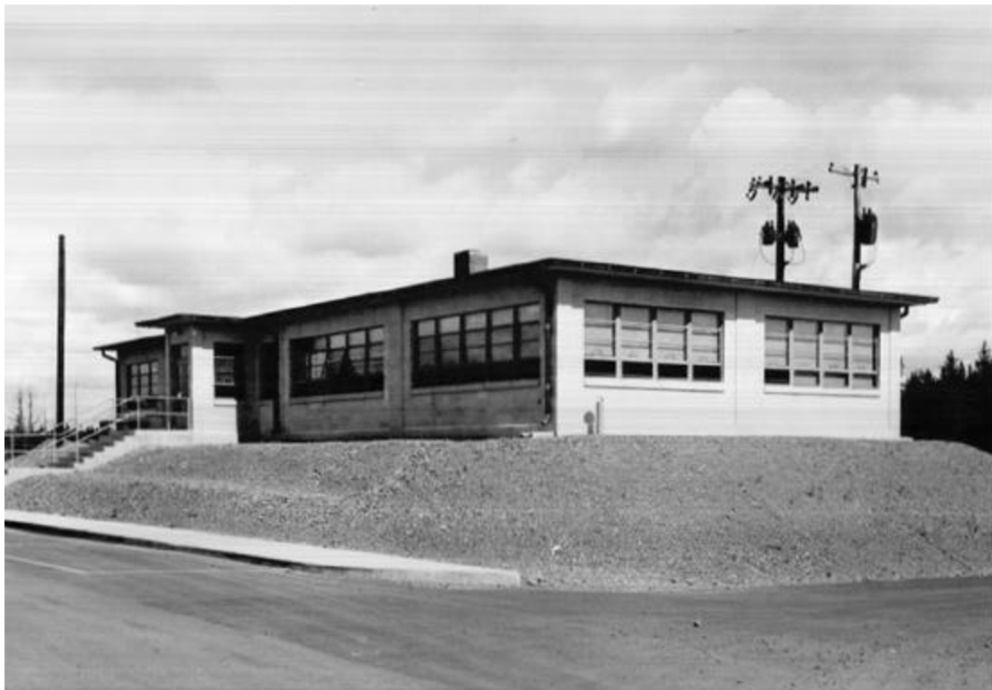
Plate 100. Black & Veatch. Command/Control Bldg. Q Area, Caribou AFS, former Loring Air Force Base. View of 1957. Courtesy, Air Force Historical Research Agency.
